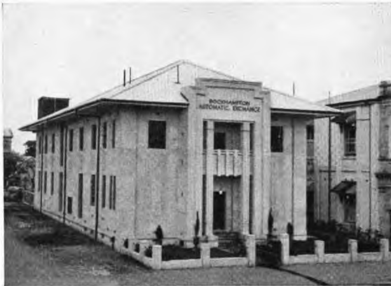
This exterior view shows the modern two-story building in which the equipment is installed.
