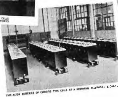
TWO BATTERIES OF SWH TYPE ALTON CELLS AT A LARGE CITY TELEPHONE EXCHANGE
