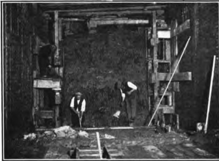
FIG. 6.—TUNNEL UNDER CONSTRUCTION.
