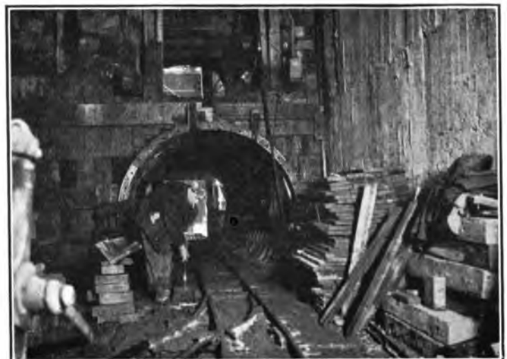
FIG. 7.—NEW TUNNEL CUT UNDER P.O. MANHOLE.
