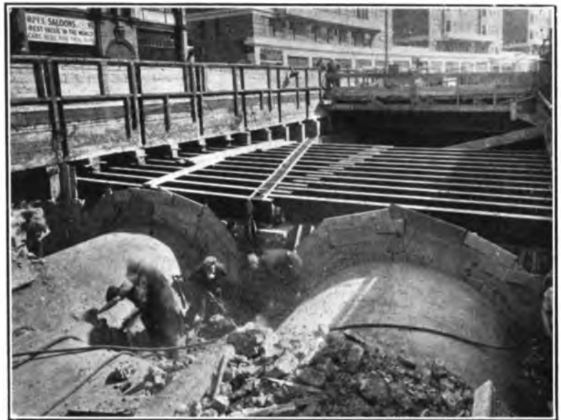
FIG. 3.—WORK IN PROGRESS OVER EXISTING TRACK.
