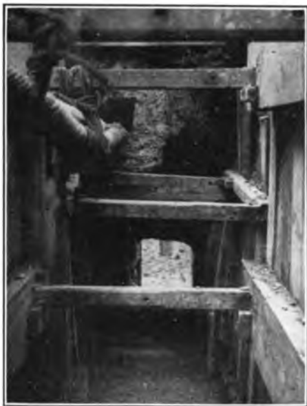
FIG. 3.—TUNNELLING UNDER SEA WALL.
