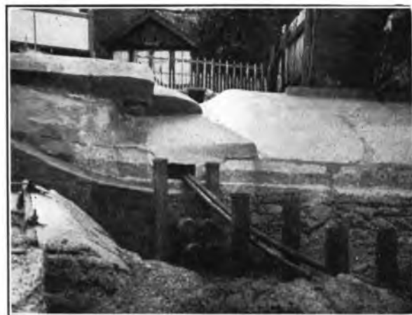
FIG. 4.—NEW PIPES IN POSITION.
