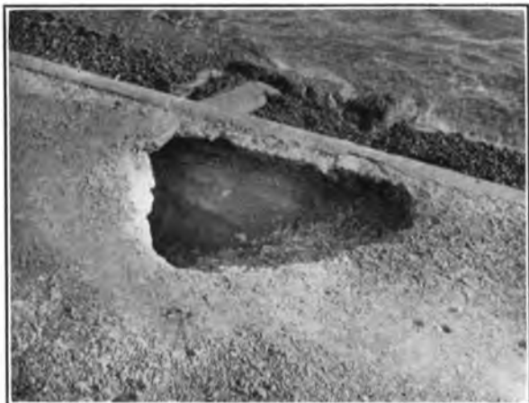
FIG. 1.—FOOTWAY SUBSIDENCE.
