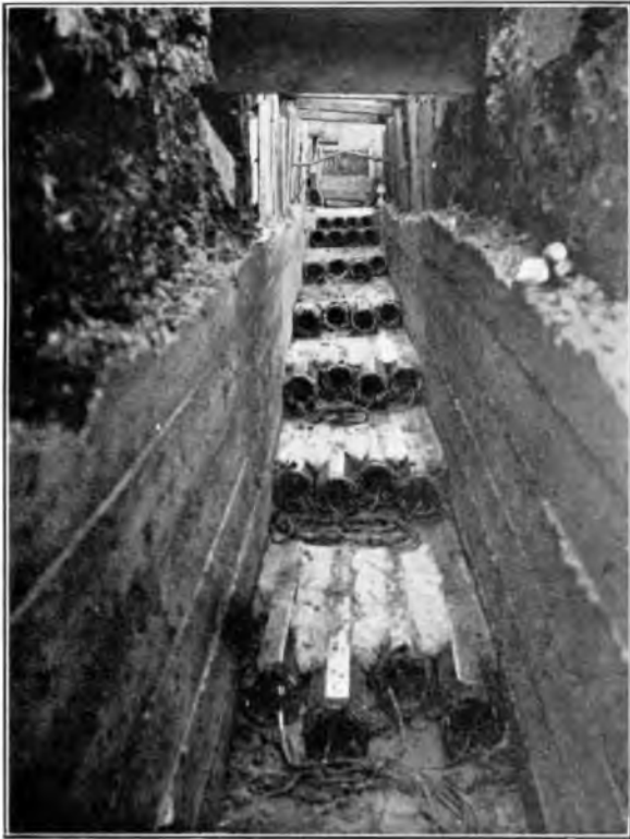
FIG. 3.—DUCT LAYING IN OPEN TRENCH IN HANOVER SQUARE.
