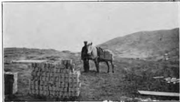
FIG. 1.—HORSES CARRYING BRICKS TO SITE.
