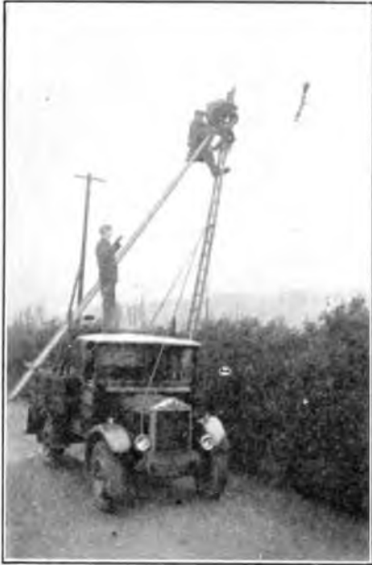
FIG. 10.—DERRICK USED TO ERECT AERIAL CABLE
