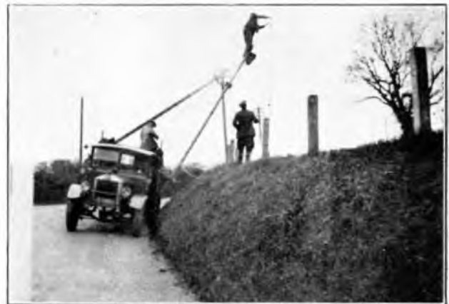
FIG. 6.—DERRICK USED WITH MAXIMUM OVERHANG.
