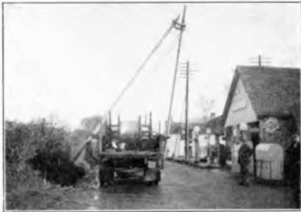
FIG. 1.—THE LADDER DERRICK
