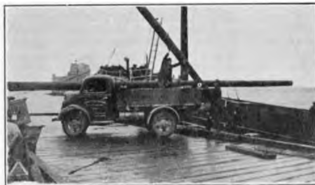
FIG. 2.—UNLOADING POLES AT BARRA.
