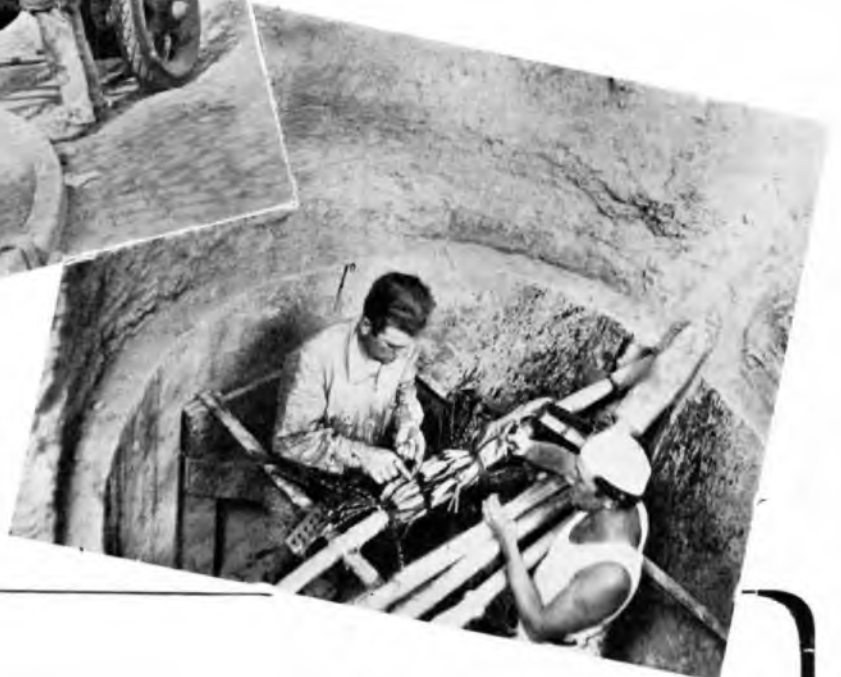
Joining operations in progress.
