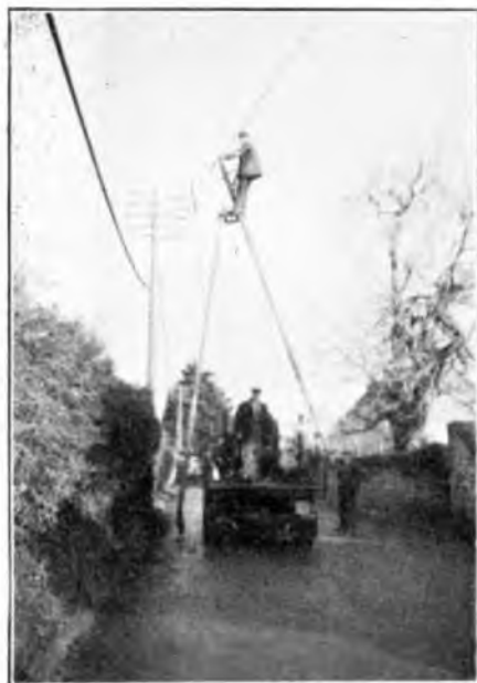
FIG. 7.—DERRICK USED IN VERTICAL POSITION.
