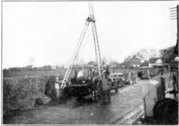
FIG. 4.—ERECTION OF DERRICK.
