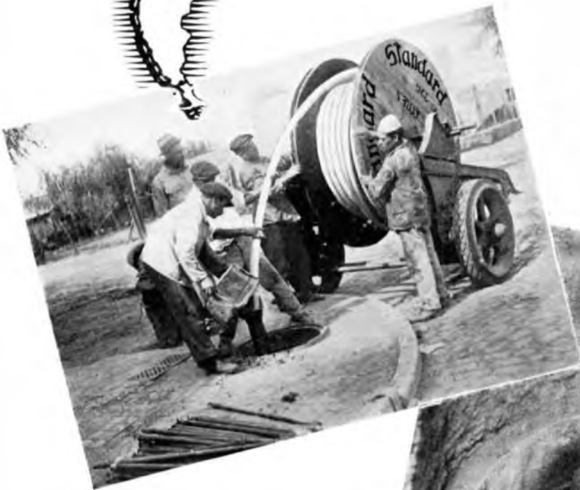
Lead-covered Cable about to be drawn into duct.
