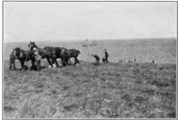
FIG. 1.—HAULING THE CABLE TO THE HEADLAND.
