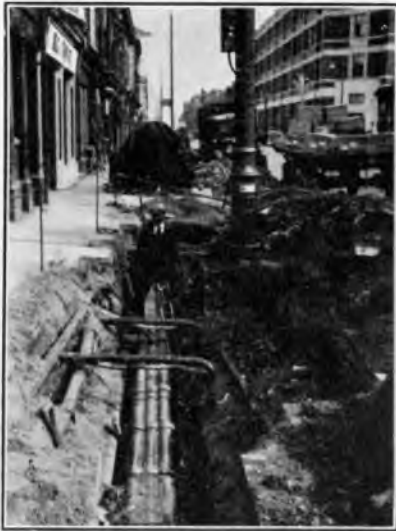
FIG. 2.—COMPLETION OF REPAIRS TO DUCT.
