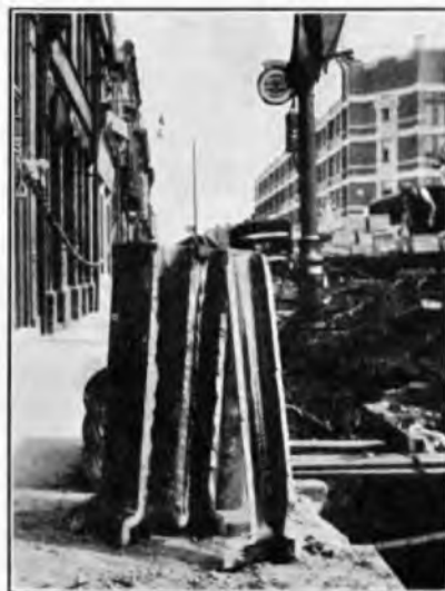
FIG. 1.—THE SPLIT 9-WAY DUCT.
