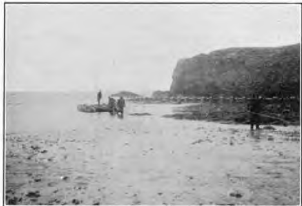
FIG. 2.—LANDING THE CABLE FROM THE RAFT.
