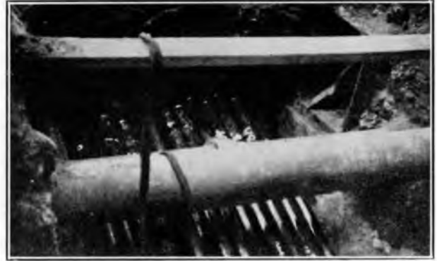
FIG. 2.—PIPES FINALLY IN POSITION.
