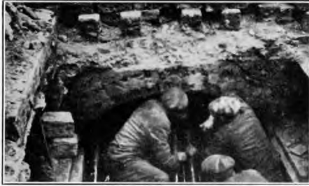
FIG. 1.—LAYING THE LAST PIPE.
