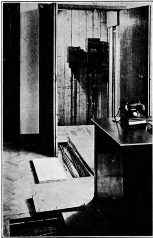
FIG. 6.—FLOOR TRENCHING.
