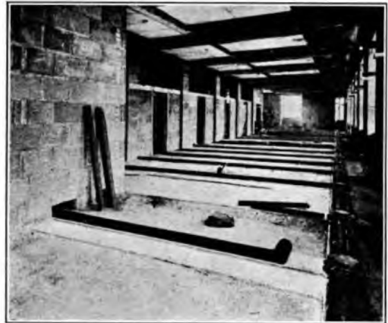
FIG. 5.—LAYOUT OF UNDERFLOOR FIBRE DUCTS.
