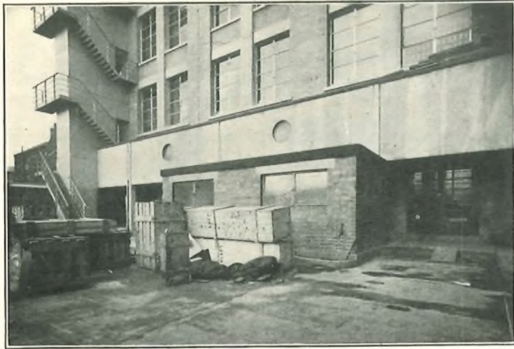
FIG. 10.—EXTERIOR OF CABLE CHAMBER.
