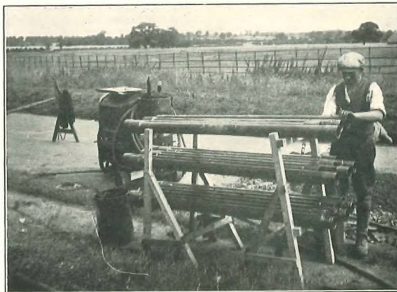
FIG. 4.—JOINTING COMPOUND BEING APPLIED.
