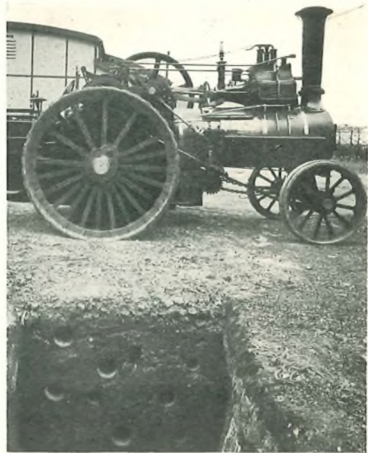
FIG. 7.—TRACTOR STANDING ON ASBESTOS-CEMENT DUCTS.
