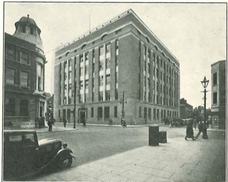
FIG. 4.—TELEPHONE HOUSE, BELFAST.
