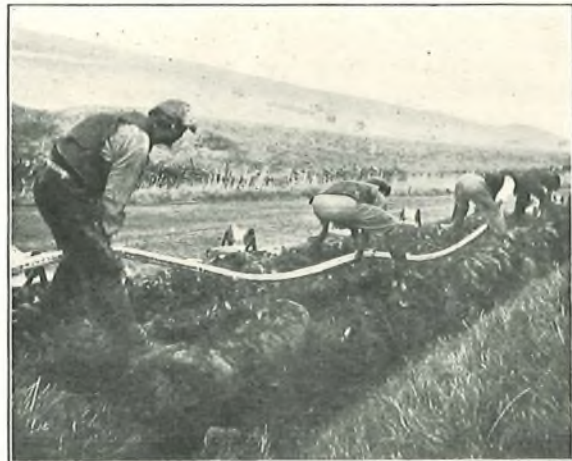
FIG. 4.—LIFTING THE CABLE INTO THE TRENCH.
