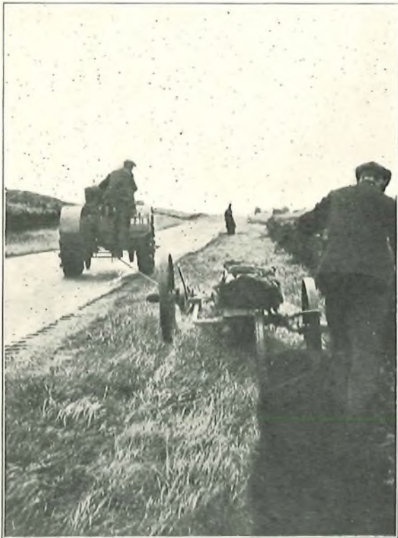
FIG. 2.—PLOUGHING THE TRACK.
