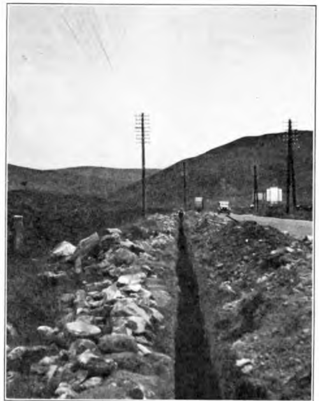
FIG. 9.—TRENCH EXCAVATION NEAR BEATTOCK.
