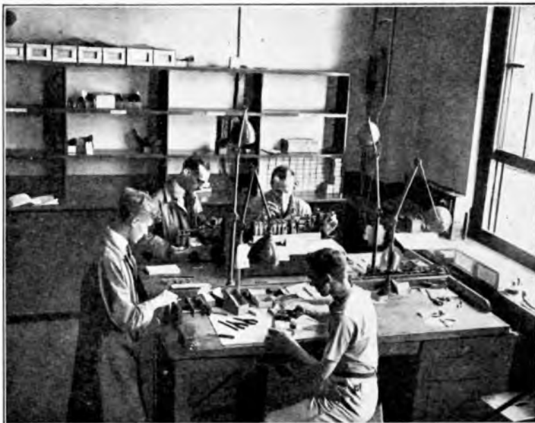
8.—ADJUSTING RELAYS, LONDON DEPLACEMENT DEPOT.
