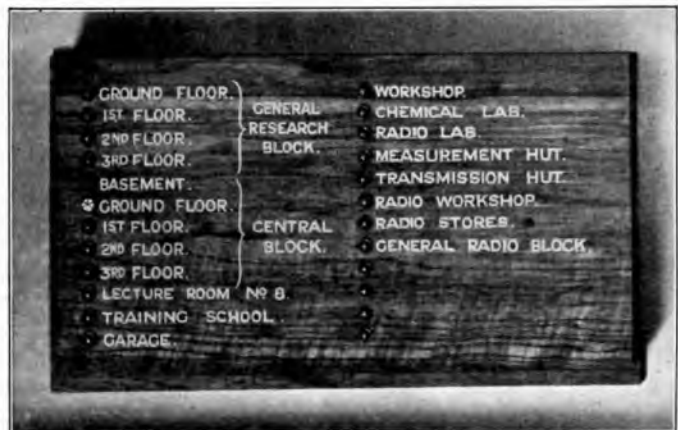
FIG. 14.—FIRE ALARM INDICATOR BOARD.
