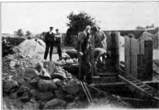
FIG. 12.—NATURE OF SUB-SOIL AT MANHOLE EXCAVATIONS.
