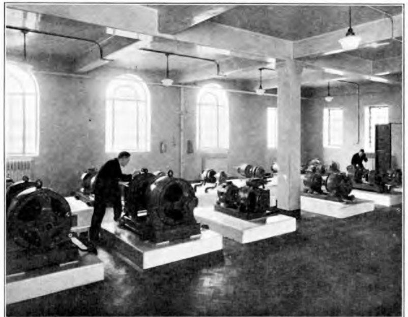
FIG. 3.—GENERATOR ROOM—CENTRAL BUILDING.
