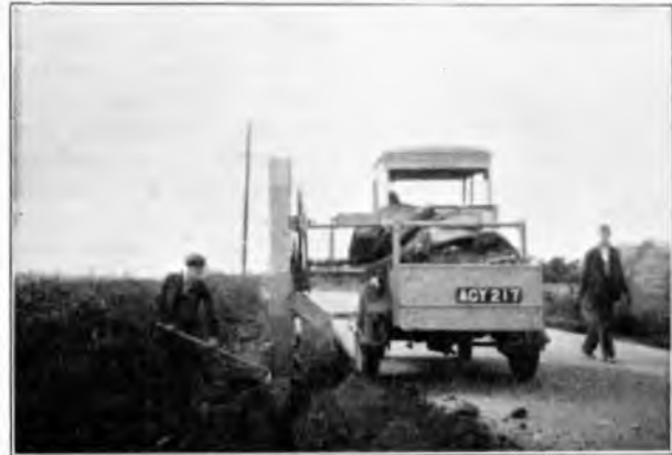
FIG. 14.—TRENCH EXCAVATING MACHINE.
