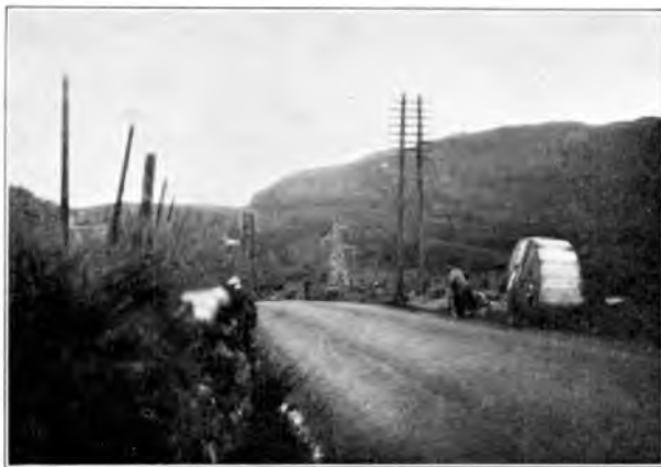
FIG. 8.—SHAP FELL, SHOWING GRID LINE.
