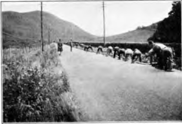
FIG. 10.—CABLEING IN PROGRESS NEAR BEATTOCK.
