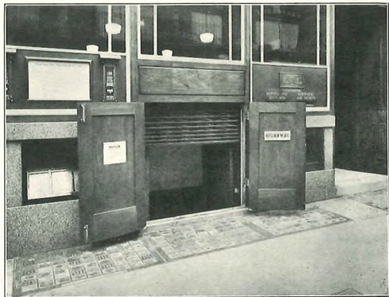
FIG. 3.—LOWER ENTRANCE TO LIFT.
