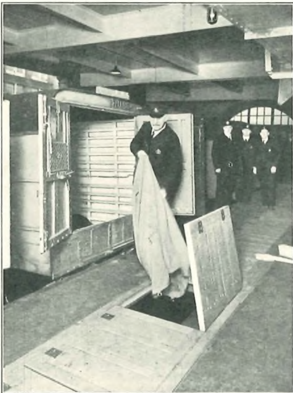
FIG. 1.—LOADING PLATFORM CONVEYORS.
