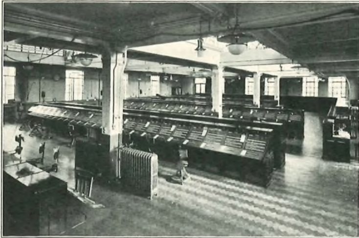
FIG. 4.—TANDEM SWITCHROOM, 1927.
