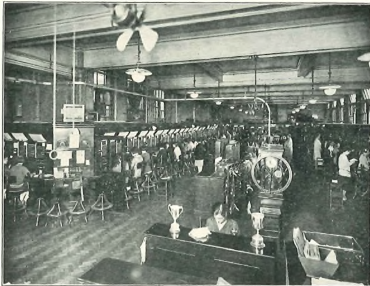
FIG. 5.—THE OLD TRUNK SWITCHROOM.
