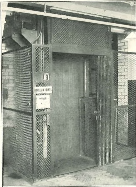
FIG. 4.—VIEW OF PAVEMENT LEVEL ENTRANCE.
