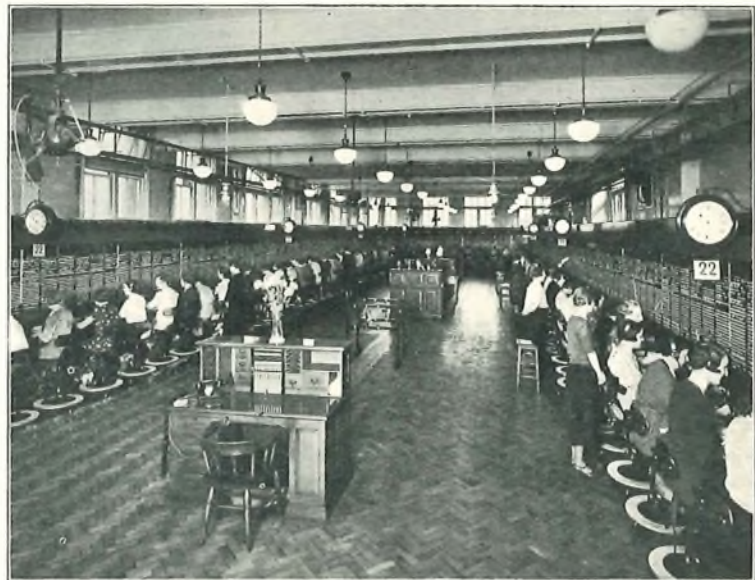
FIG. 6.—THE NEW MAIN TRUNK SWITCHROOM.
