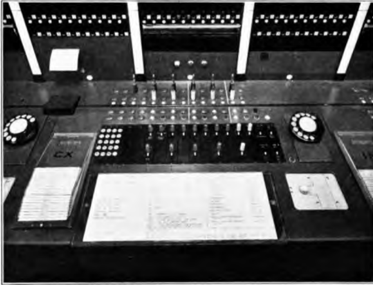
FIG. 2.—DESPATCH AND DISCHARGE VALVES ON TICKET TUBES AT OPERATOR'S POSITION.
