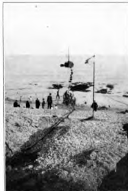
FIG. 7.—PREPARING TO HAUL THE CABLE UP THE BEACH.
