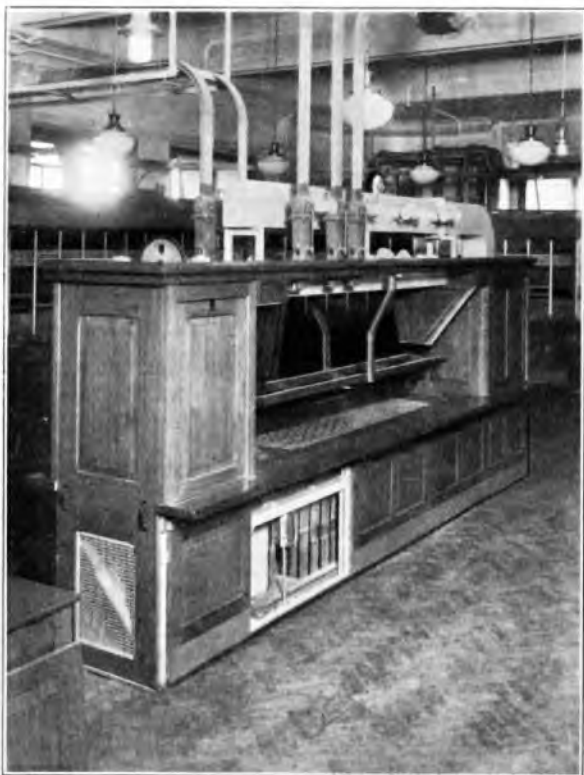
FIG. 5.—P.D.P. FOR INLAND TRUNK EXCHANGE AS EQUIPPED ORIGINALLY WITH MIX AND GENEST TERMINALS.
