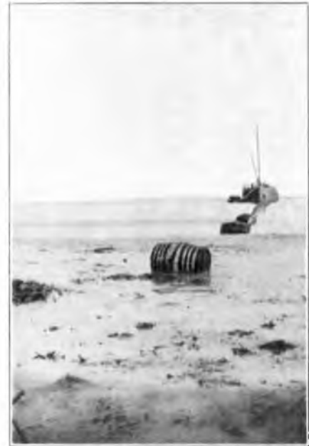
FIG. 4.—FLOATING THE CABLE ASHORE AT ST. MARGARET'S BAY.
