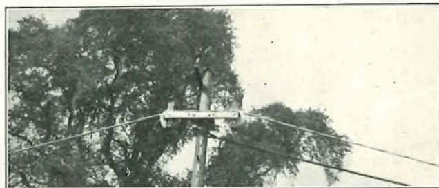
FIG. 3.—CABLE SHEAVES SECURED TO POLE.
