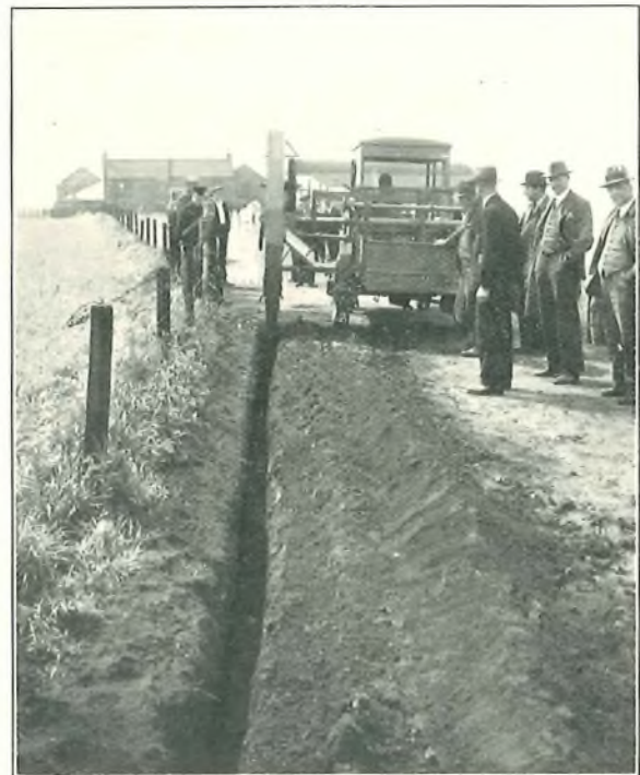
FIG. 2.—TRENCH EXCAVATOR IN ACTION.
