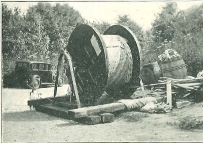
FIG. 4.—CABLE DRUM AND BRAKE.
