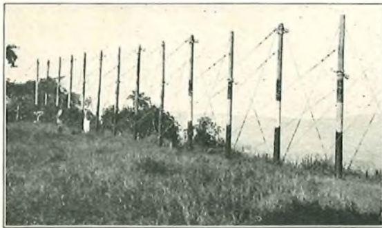
FIG. 14.—TERMINAL OF SPAN CROSSING BRAHMAPUTRA RIVER.
