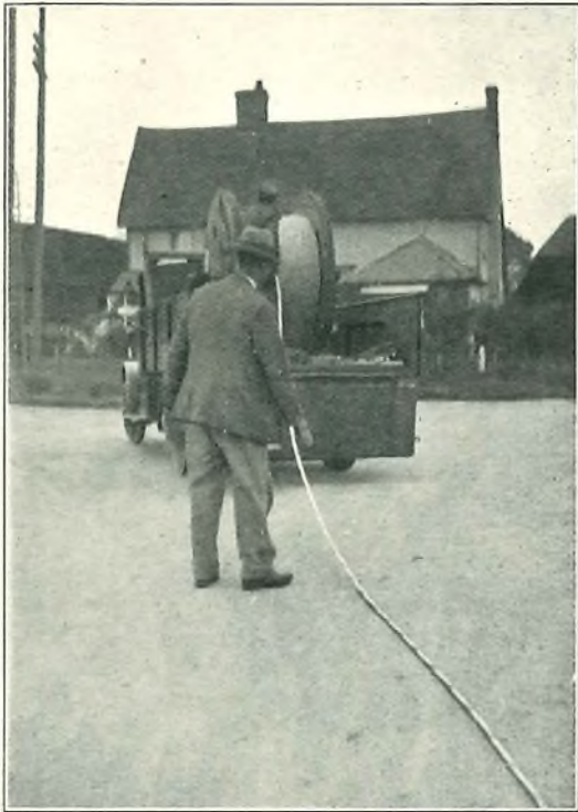
FIG. 6.—PAYING OUT CABLE FROM LORRY.
