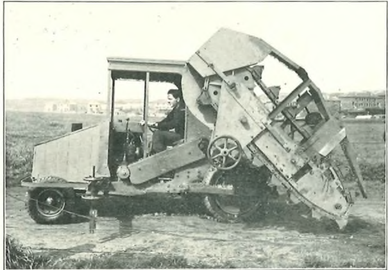
FIG. 1.—MECHANICAL TRENCH EXCAVATOR.
