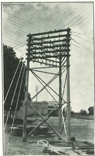
FIG. 7.—TRIPOD TERMINAL CDE POSTS.
