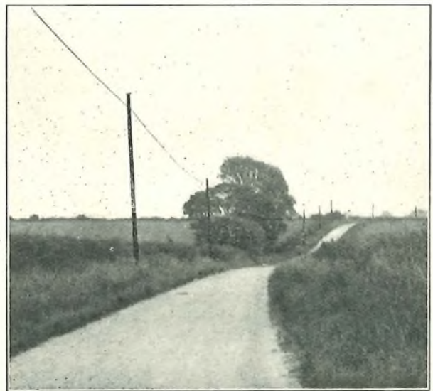
FIG. 8.—A SECTION OF CONTINUOUSLY SUSPENDED AERIAL CABLE.
