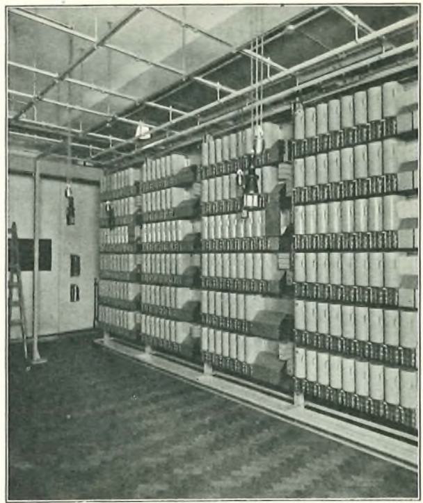
FIG. 5.—FINAL SELECTORS, CENTRAL EXCHANGE.
