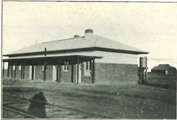
FIG. 4.—REPEATER STATION BUILDING: TRANSCONTINENTAL ROUTE.
