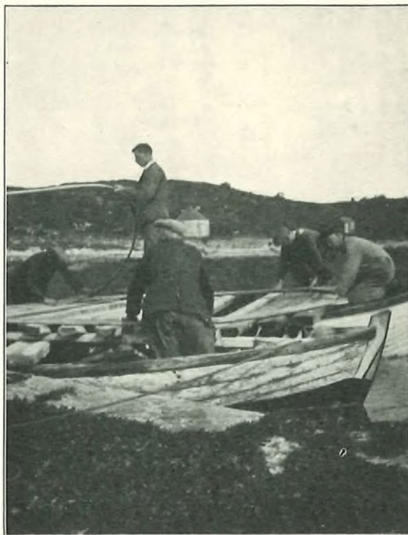
FIG. 2.—COILING THE CABLE.
