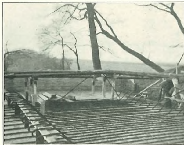
FIG. 1.—PIPES SUPPORTED ON SHUTTERING.
