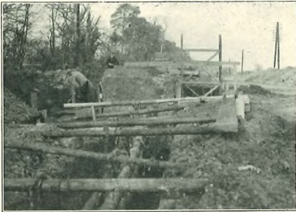
FIG. 1.—MANHOLE READY FOR LOWERING.
