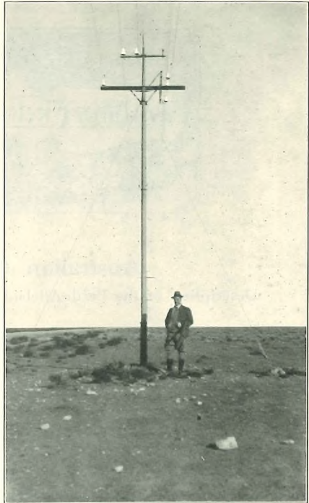
FIG. 2.—TYPICAL TRANSPOSITION POLE.
