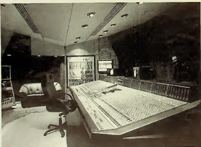
Control room Studio 1 with SL 9072-J console
