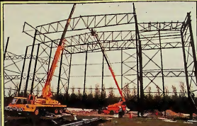
Work in progress: the conversion takes place
