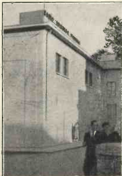
The studio building at the foot of Monte Bré, in Lugano.
