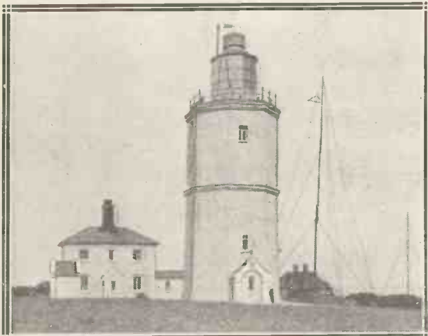
Another radio station that handles a large ship-to-shore traffic is the G.P.O. transmitter situated at North Foreland. It recently had its spark set replaced by the most up-to-date "I.C.W." equipment. The high tower in the foreground is the famous North Foreland lighthouse.
