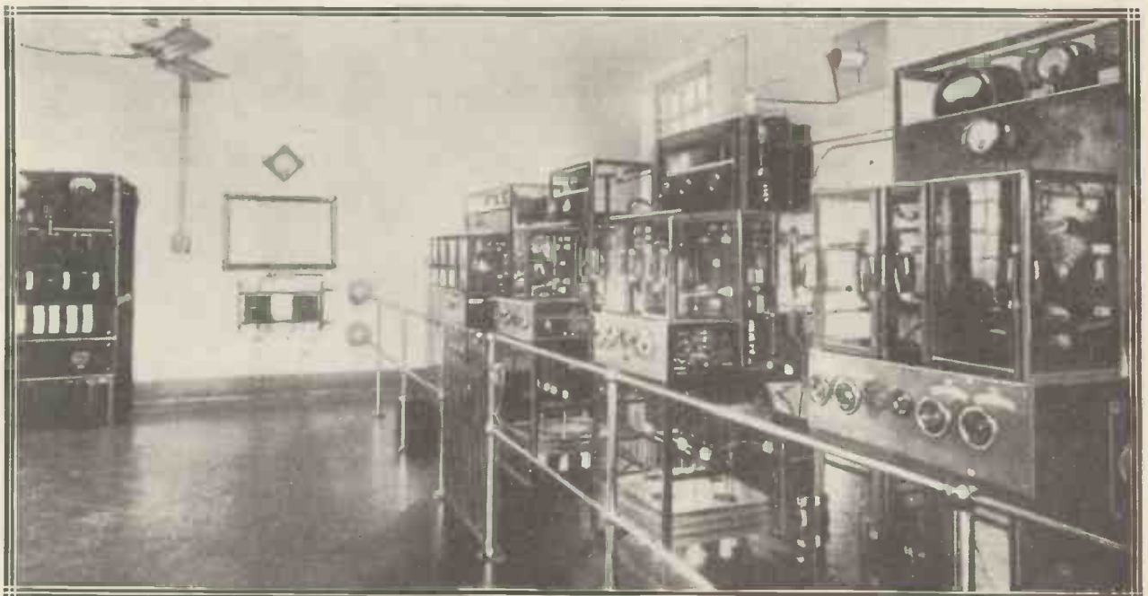
A view of the 12-kw. Marconi G Type transmitter that has recently been installed at Bombay.
