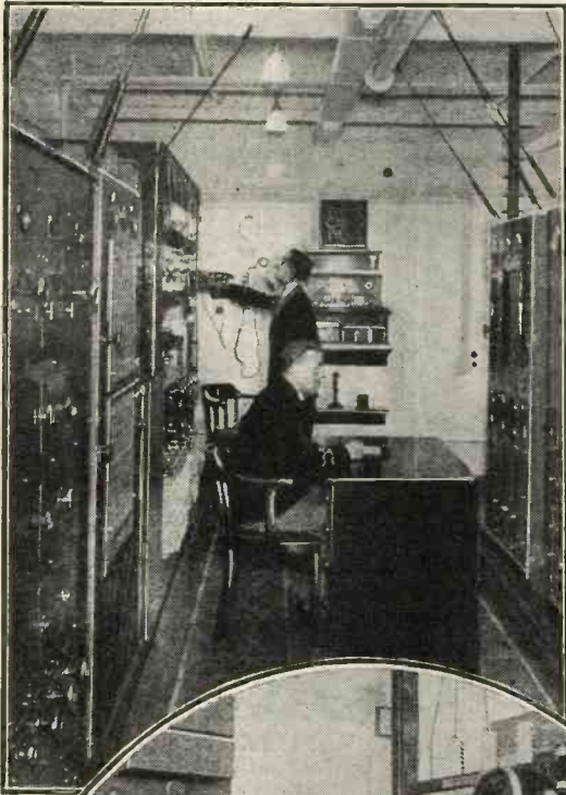
A short-wave telegraph transmitter and receiver is shown to the right, and a band repeater amplifying equipment to the left.
