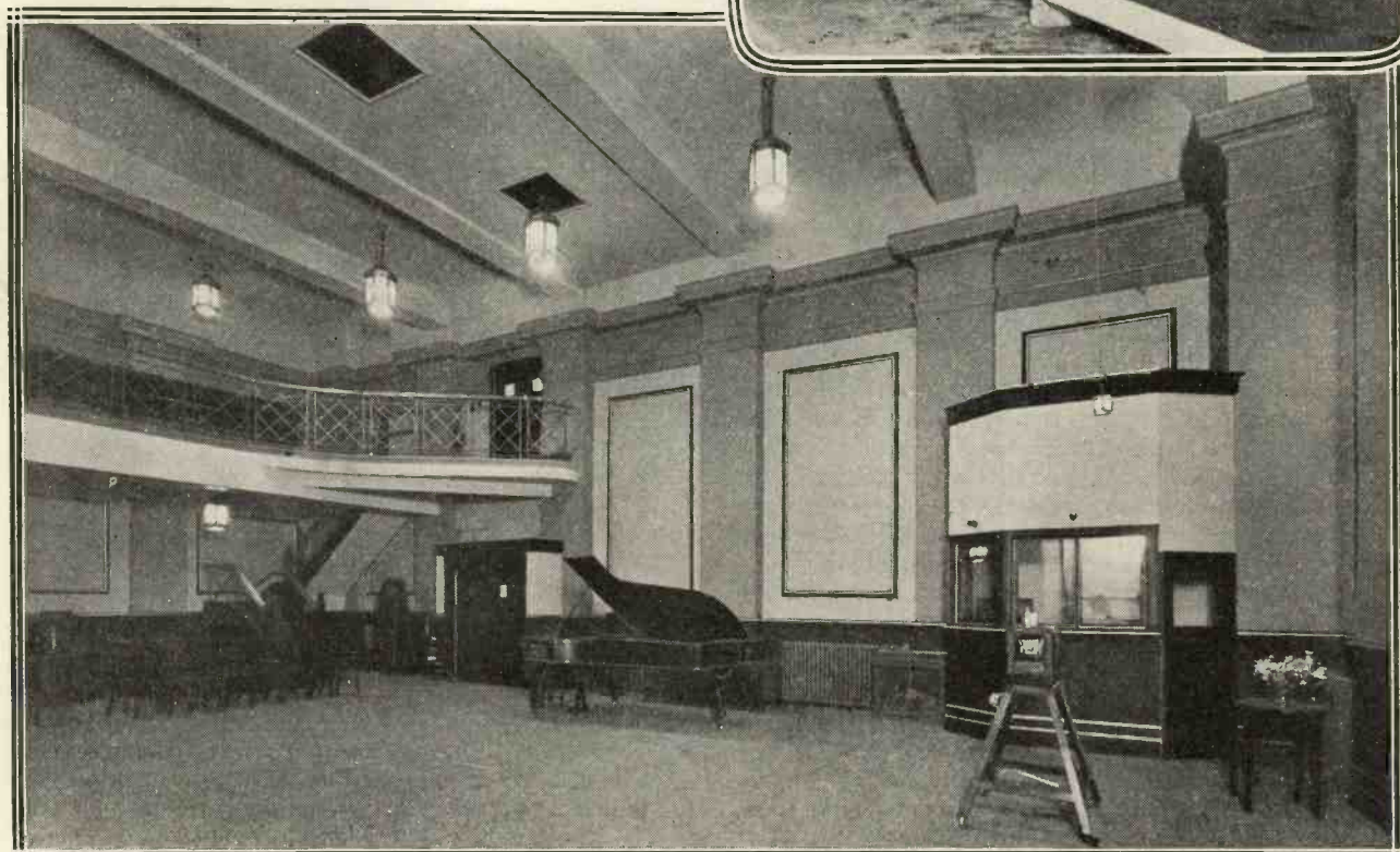
Workmen are shown cementing the floor of the gallery of one of the giant studios in the upper picture. Below it is a view of the main Manchester studio. Note the Announcer's box on the right.
