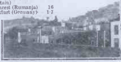
The Station at Funchal works on 47 metres.
