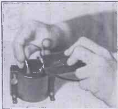
The continuity of a transformer's windings can be tested with a small battery and a pair of 'phones.
