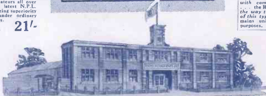
Here is shown the new R.I. Factory and Offices.
