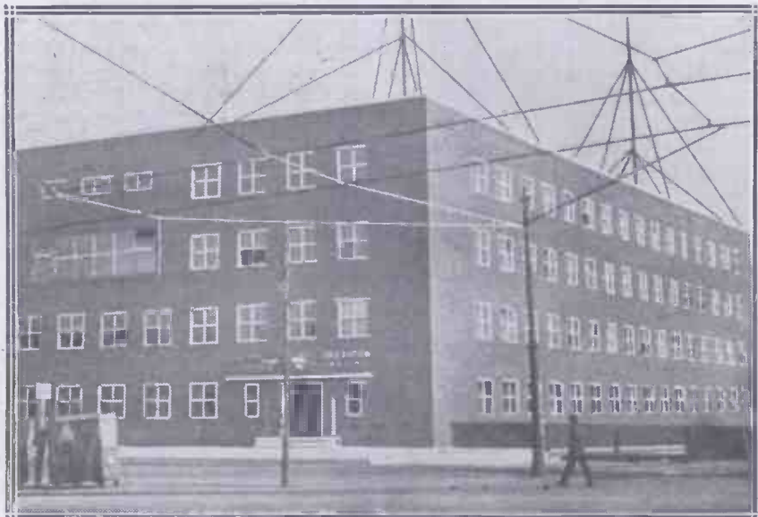
A Berlin radio building in which immense pains have been taken with screening to prevent pick-up and interference
