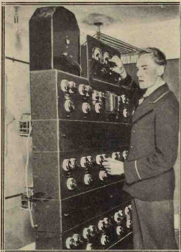
The set shown here is installed in Baker Street, London, and supplies two hundred families with loud-speaker programmes.
