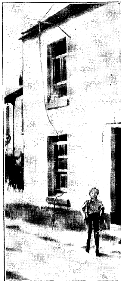
This listener has taken his earth lead right through the pavement.
