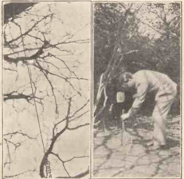
To the left is shown the method of clipping the aerial in position, and the right-hand photograph shows the making of an efficient earth connection.
