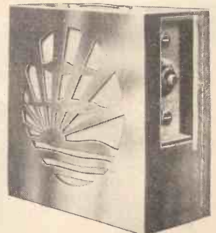
The "Pye" portable has its controls on a small panel in the side of the case.
