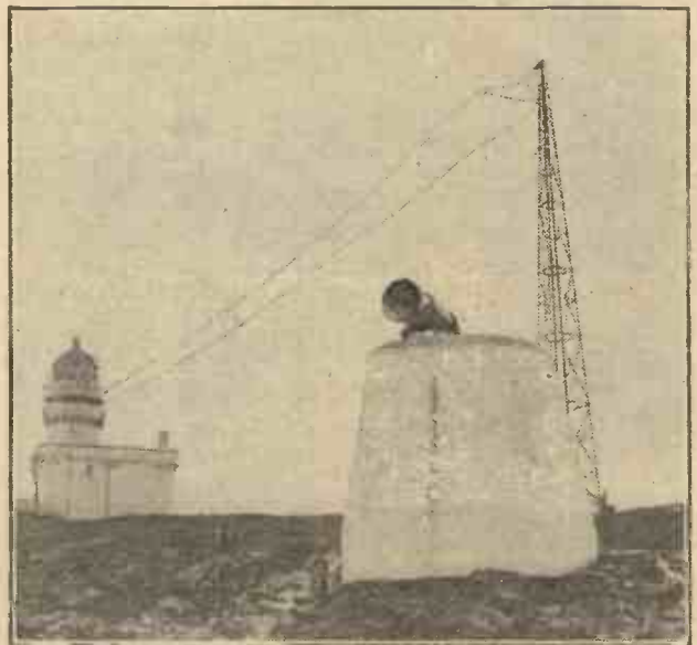
This wireless beacon station, built at Fraserburgh, was the first to be built on the mainland of Scotland. Note the fog siren in the foreground.
