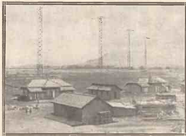
A view of India's Beam transmitting station at Poona, showing four of the five 275-ft. masts.
