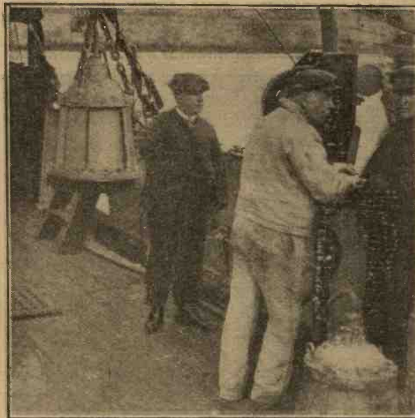
Heaving up the submarine oscillator which is used in conjunction with the wireless beacon for direction finding at sea.
