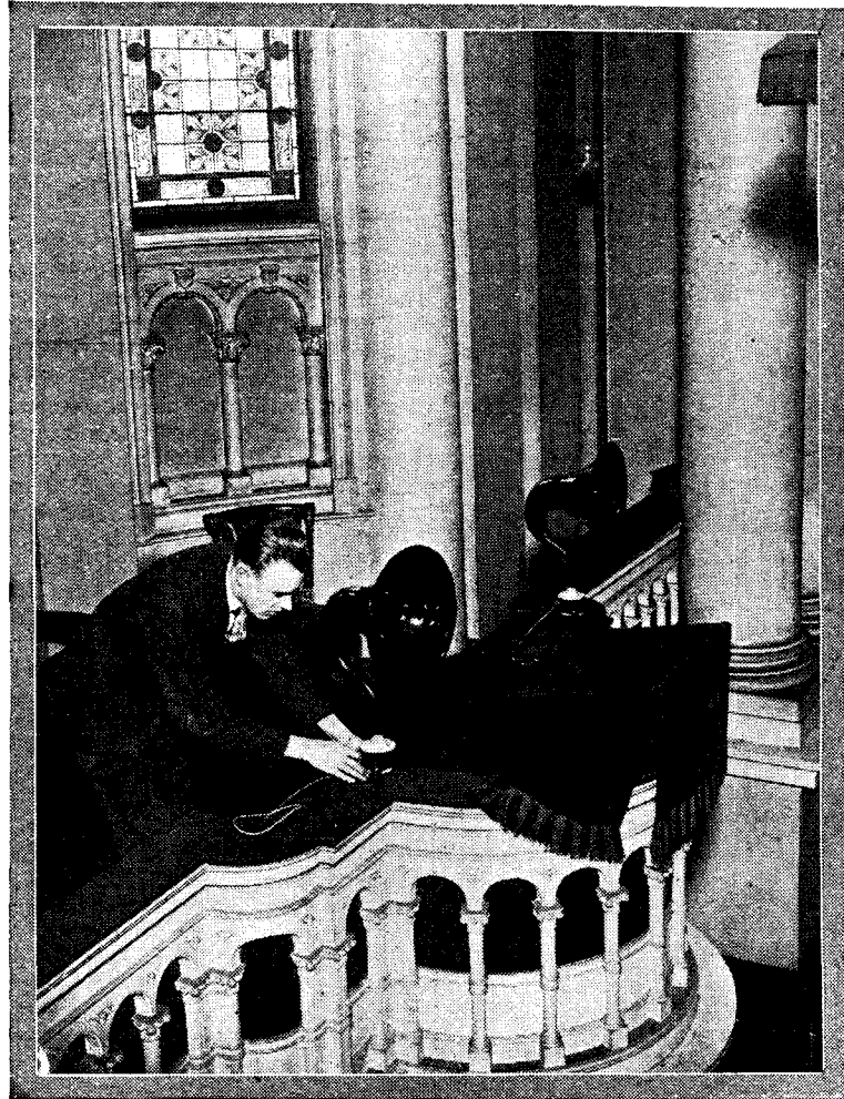
Arranging loud-speaker horns ready for broadcasting a Good Friday service from 2LO to the congregation of Hinde Street Wesleyan Church, London.
