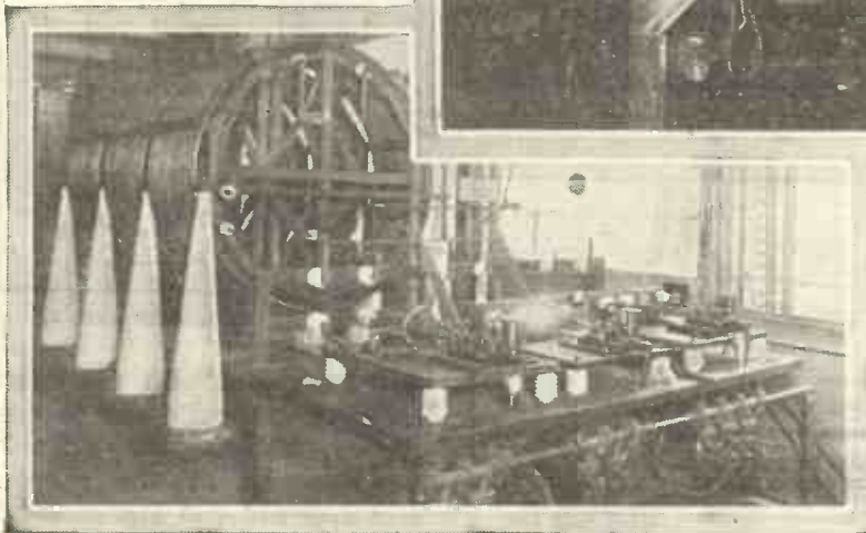
Below: The Creed signalling switch and aerial loading coil.
