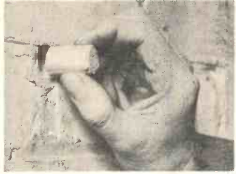
Fig. 4. —INSERTING THE PLUG.
