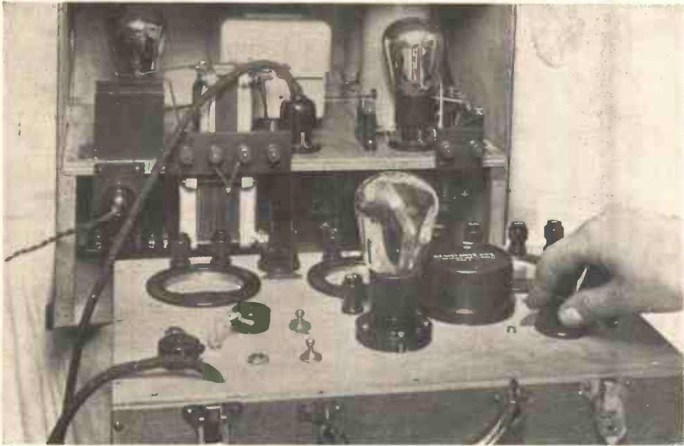
Fig. 4.—TESTING THE DETECTOR VALVE OF THE TWO-STAGE SET DESCRIBED ON P. 841.
