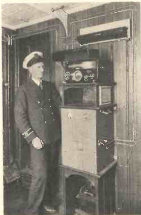
Fig. 1.—THE MARCONI ECHOMETER SOUNDING DEVICE FITTED TO S.S. Pennyworth .
