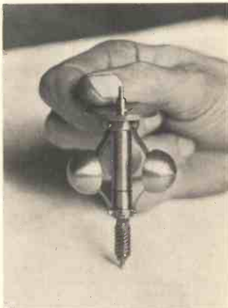
Fig. 2.—DETAILS OF THE GOVERNOR.
