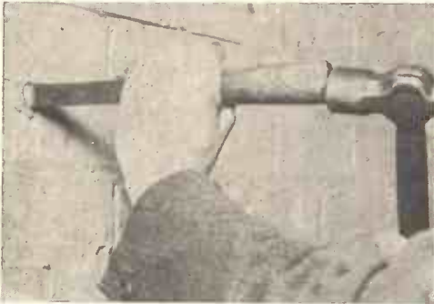
Fig. 5. —SPLITTING THE PLUG WITH A CHISEL.
