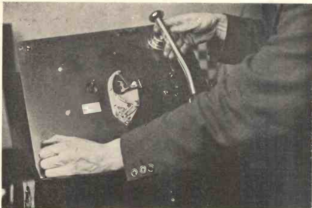
Fig. 9. —LIFTING OFF THE MOTOR BOARD.
