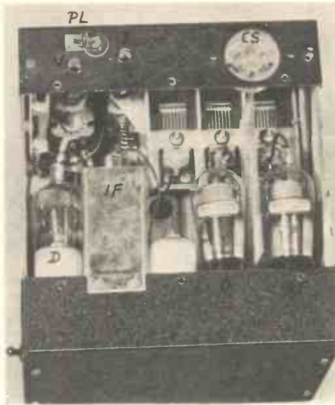
Fig. 3.—FRONT ELEVATION WITH FRONT COVER REMOVED. ALL MODELS.
