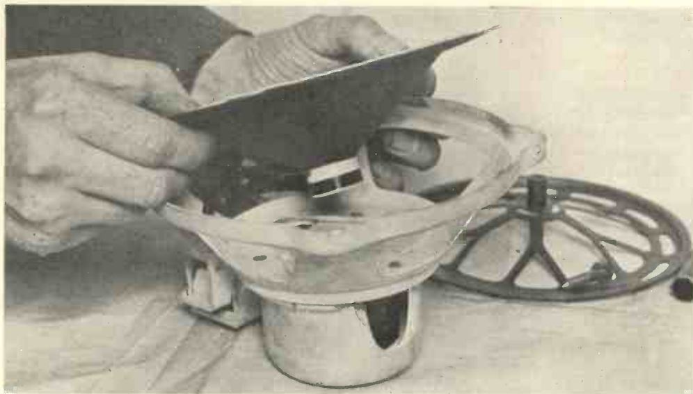
Fig. 23.—LIFTING OUT THE DIAPHRAGM AND COIL OF A MAGNAVOX SPEAKER.
