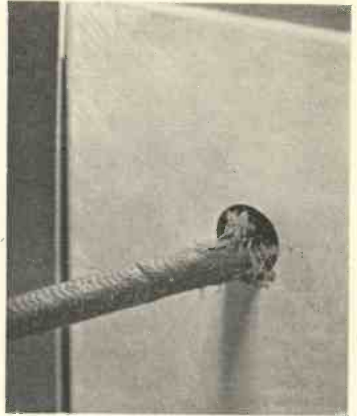
Fig. 3. —THE INCORRECT WAY OF MAKING A HOLE IN A METAL CASE.
