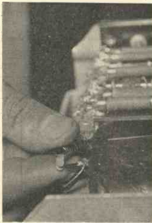
Fig. 17. —FITTING A MAINS TRANSFORMER FUSE REPLACEMENT.
