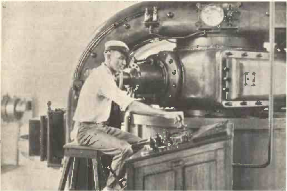
Fig. 1. —AN ARC GENERATOR OF 500 K.W. INSTALLED AT CAVITE, PHILIPPINE ISLANDS.
