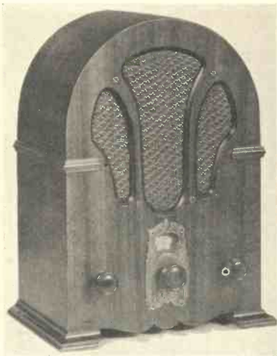
Fig. 16.—RCA VICTOR MODEL R.5. A four-valve tuned radio-frequency receiver.
