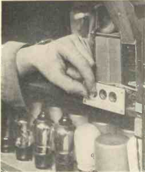
Fig. 17.—FITTING NEW FUSE BULB TO CORRECT TAPPING FOR MAINS SUPPLY.
