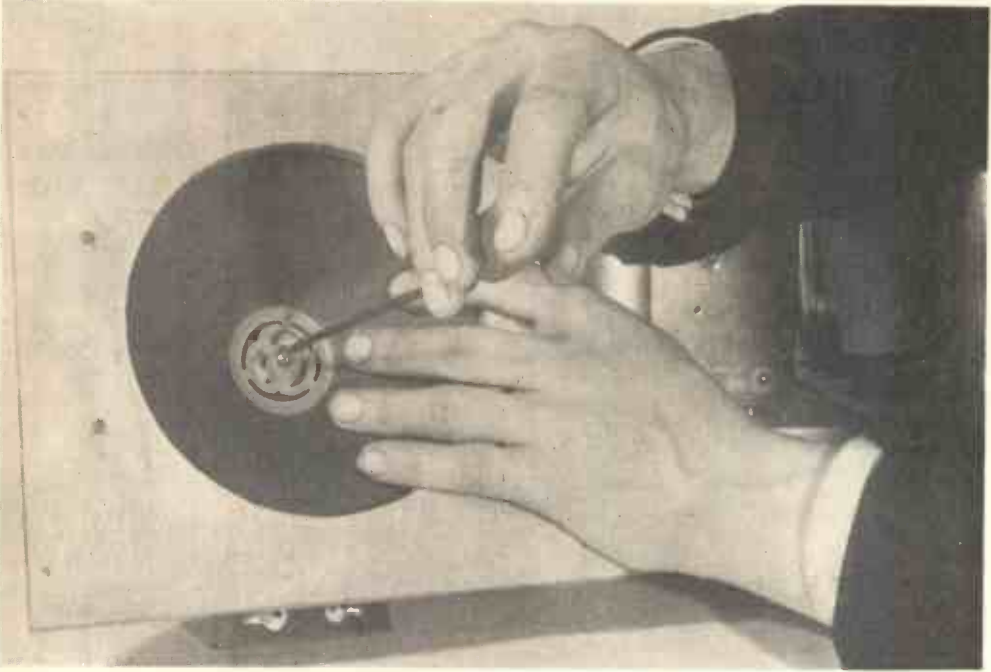
Fig. 10. —ADJUSTING THE SPEECH COIL.
