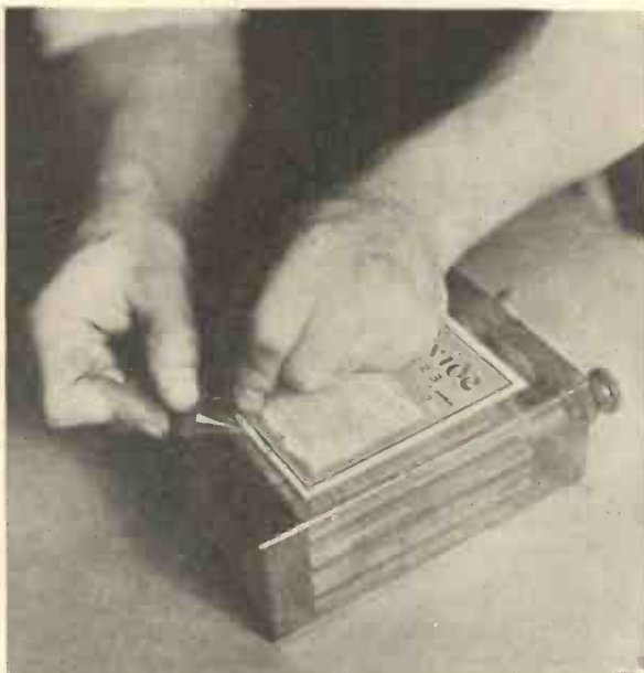
Fig. 14.—PATCHING LEAKY CELLULOID CONTAINER.
