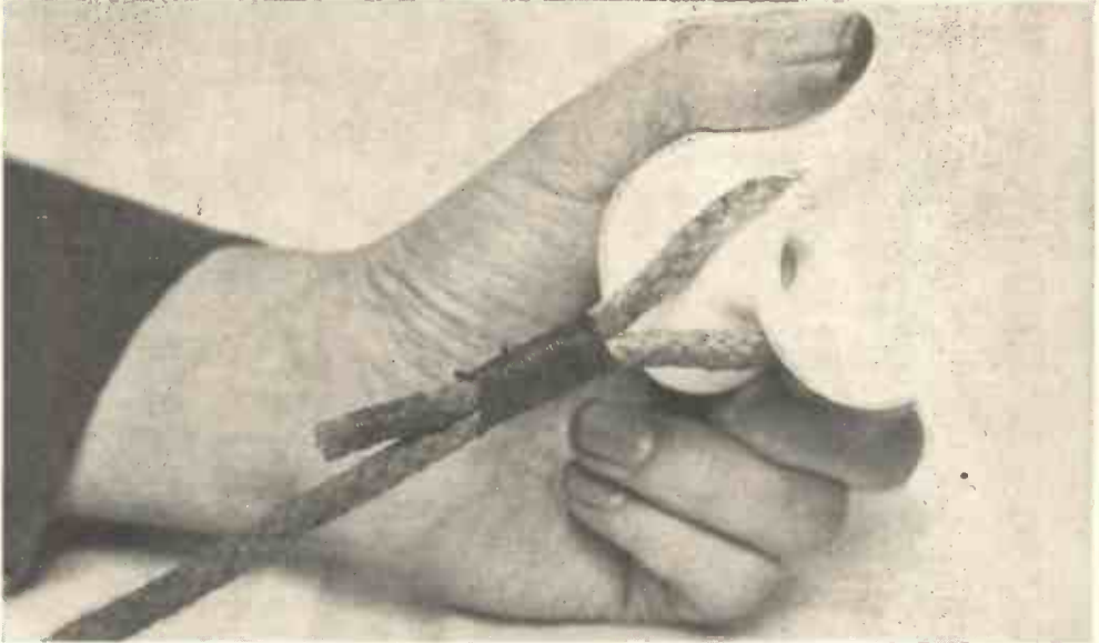
Fig. 1. —HOW TO JOIN ROPE TO THE INSULATOR.
