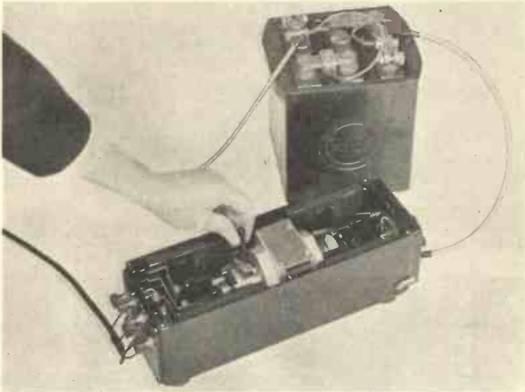
Fig. 9.—CLEANING THE COMMUTATOR OF AN ANODE CONVERTER.
