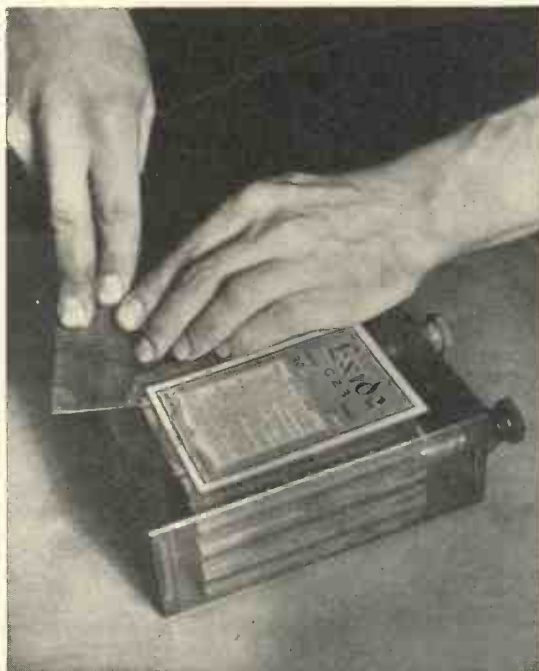
Fig. 12.—HOW TO CURE A LEAKY CELLULOID CONTAINER.
