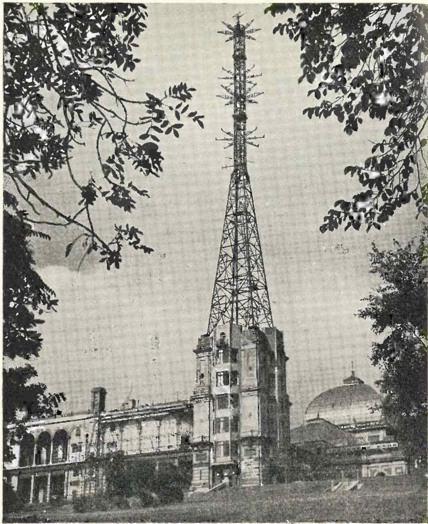
Last link in the chain of television transmission: the complicated aerial array mounted on a huge lattice mast on the North Tower of Alexandra Palace. Both sound and vision transmissions are radiated from it.
