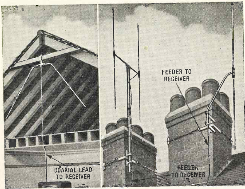
Three representative television aerials. That shown on the left is one of various types of indoor aerial suitable for use within, say, ten miles of the transmitter. The H-type aerial is the most sensitive and is also useful in reducing interference caused by motor-cars. The dipole shown on the right is completely satisfactory at distances up to about 25 miles from the TV transmitter, particularly when it is not used near to a main road.
