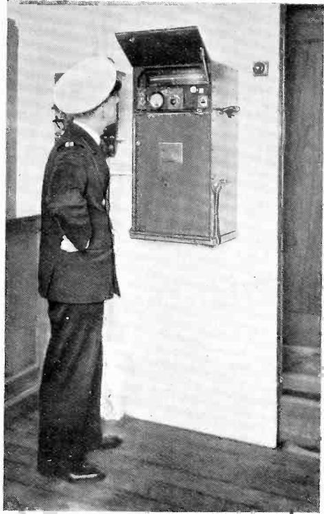
A ship's officer "taking soundings" with the Marconi Echometer.
