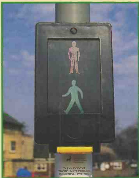
Top left: Photo 1. The kerbside sensor ensures that a pedestrian wishes to cross before the crossing controller proceeds to the pedestrian phase. An experimental infra-red sensor is also included, mounted on the top of the signal post.
