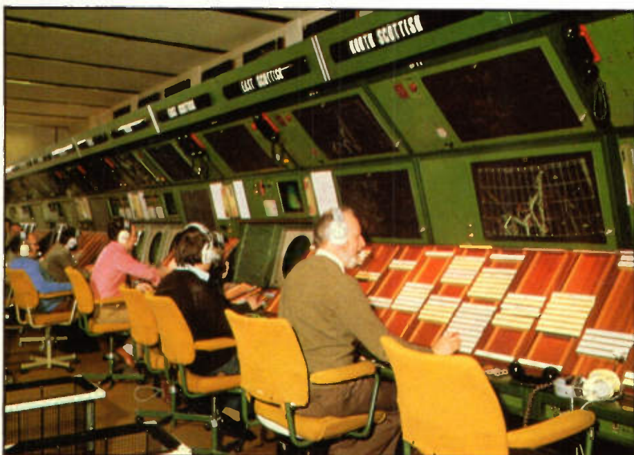
Scottish Air-Traffic Control Centre Operations Room.
