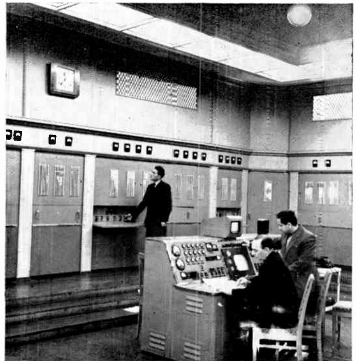
Interior view of control panel
