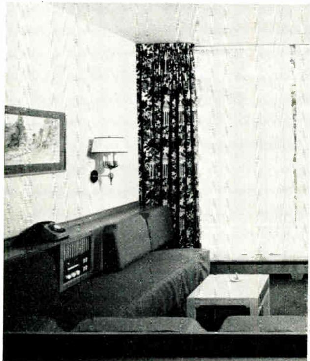
Each bedroom has a bedside panel carrying the push-button controls for the 6-channel relay television system; the controls for the closed-circuit television system linking all major parts of the hotel; the controls for the 4-programme radio service; the background music controls; the indicator for the 'message waiting' system which is combined with the key rack and ensures that a client proceeding straight to the room will see the visual indication and telephone the enquiry desk for the message; the cancel button for the labour-saving 'morning call' system whereby guests book their calls through an automatic storage unit; and light switches
