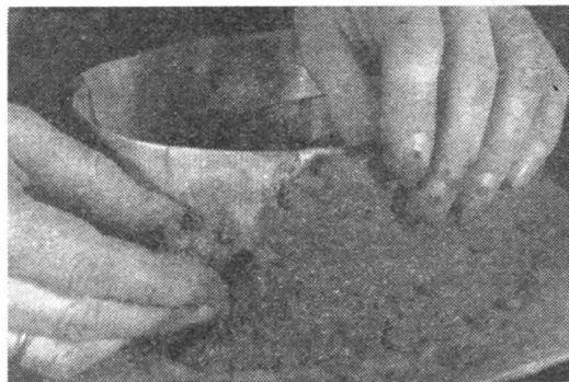
Plastering cement on aluminium mould
