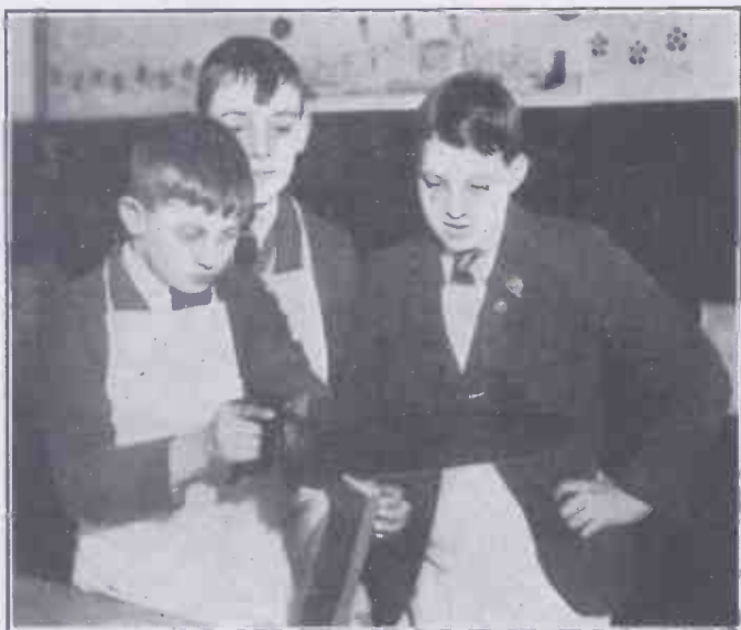
STARTING A DOWN-CUT WITH A RIPPER-SAW FOR A TENON.
