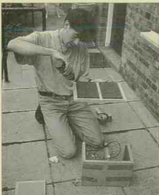
Apply an even layer of glue to the cabinet seams.
