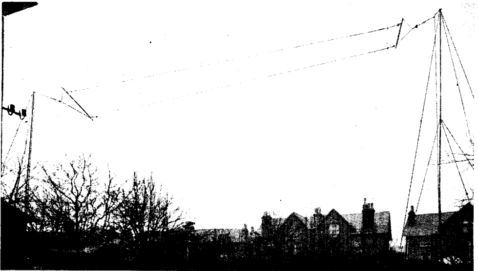
AERIAL USED FOR WIRELESS TRANSMISSION FROM 6 RJ
