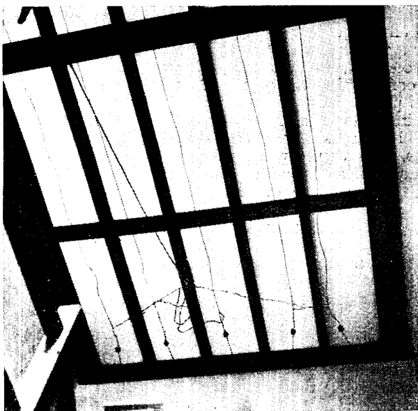
Fig. 2 (right). Over the well of a staircase this aerial is erected. Five wires, about 18 in. apart, are connected to a common lead-in. Fig. 3 (left). Screw eyes are fixed to the top edge of the picture rail to support this aerial, which consists of three or more strands stretched across the room
