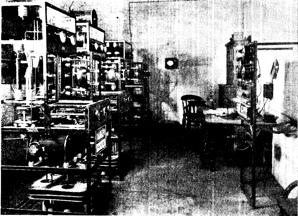
Fig. 3. Cardiff station is equipped with the Q type telephony transmitter, which is seen in the photograph. Operation is carried on in much the same way at all the B.B.C. stations, and the mechanical manipulation, control of output, modulation and methods of signalling fluctuations in strength or weakness of signals is no less an art than the actual broadcasting
