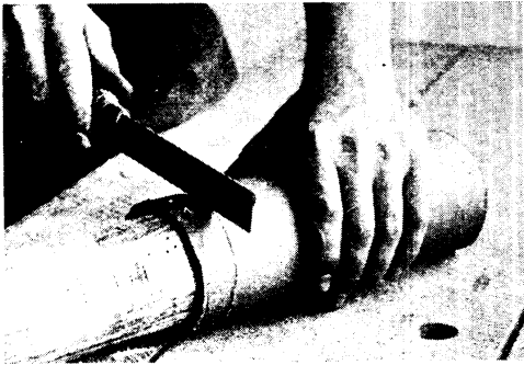
Fig. 1. By placing a wooden liner in this manner to prevent the tube buckling, a clean cut can be made with a brass-backed saw
