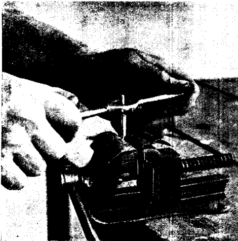
BRASS SCREW CUTTING AND TAPPING BY HAND
