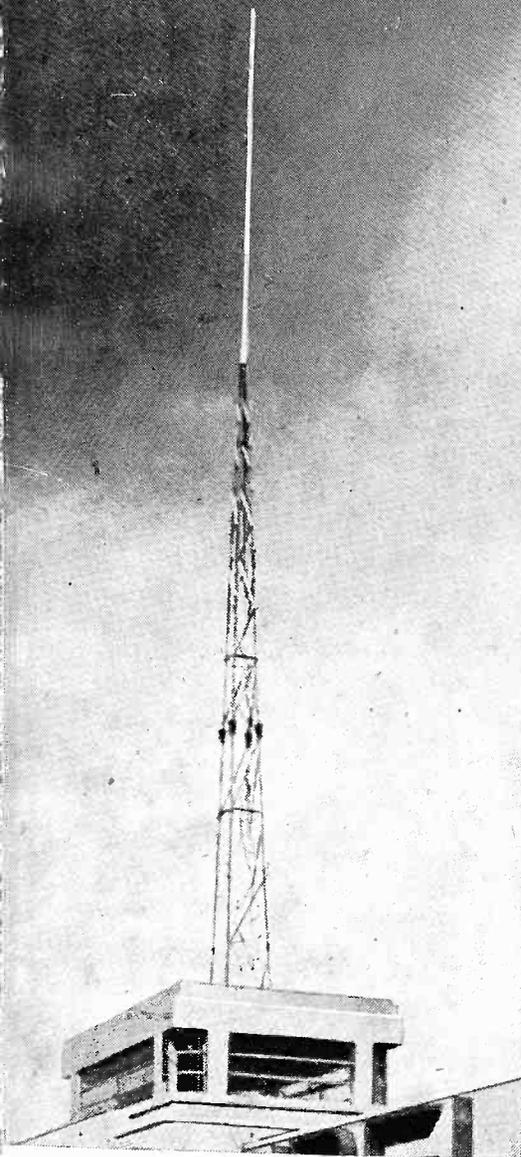
**VERTICAL AERIAL** developed for the Army offered as ideal for laboratories, factories, relay stations, etc., where serious reception is required. Porcelain insulators 15ft. from base, leaving 37ft. collector generally terminating in "Eliminoise" transformers and transmission line.
