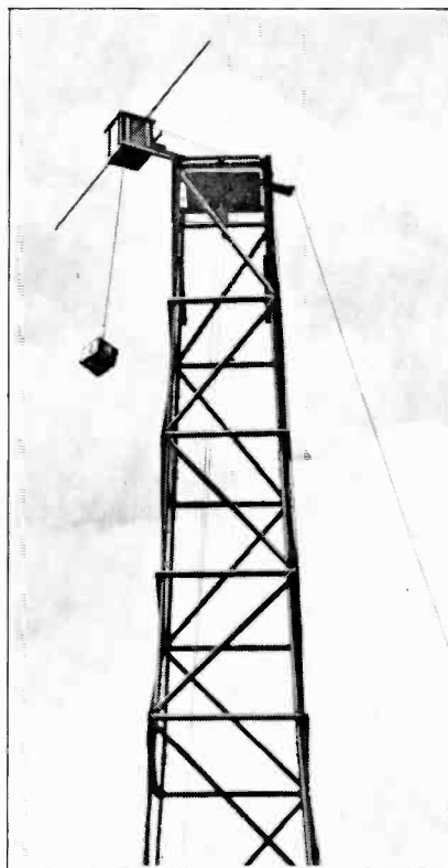
Fig. 4(b).—Close-up view of transmitter, housing and dipole aerial.
