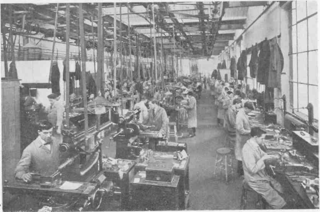
Some idea of the extent of the Sterling works can be gathered from this view of their own tool shop.
