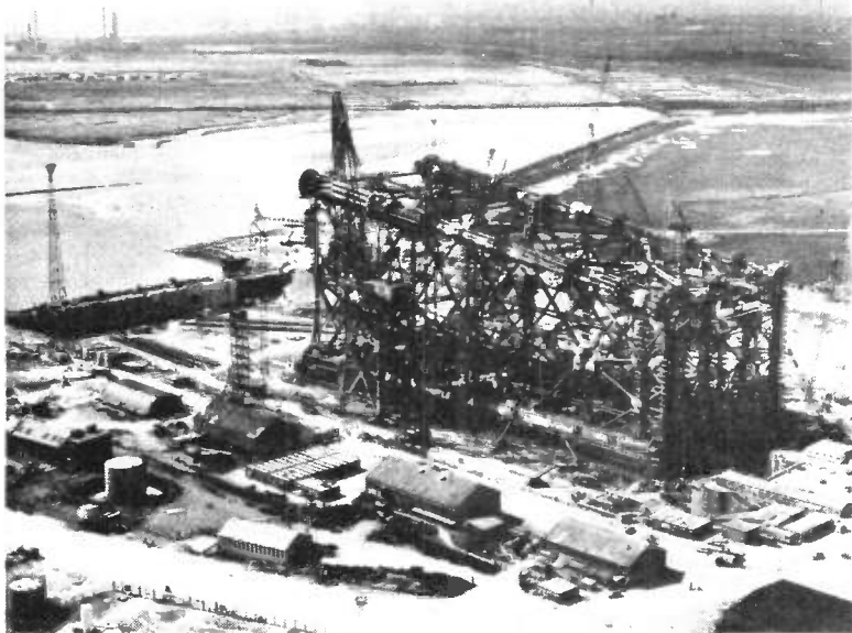
Giant 700ft high oil production platform for Burmah Oil's Thistle 'A' field under construction. It was successfully placed in position with the aid of over £1 million worth of remote control and telemetry equipment of EMI design.
