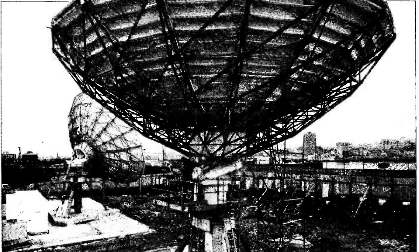
The new generation — Aerials 1 and 2 (undergoing installation) in the London Docklands.
