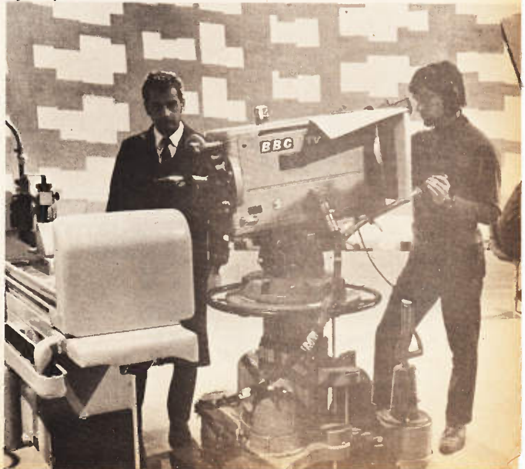
The portable version of the most advanced broadcast television camera, the Marconi Mark VIII. The camera is designed to produce high quality pictures which can be inter-cut with pictures from other studio cameras without degradation of picture quality. The Mark VIII Portable, which can be connected to a standard camera control unit, retains the features of automatic alignment and colour balance, particularly important for portable cameras which are subjected to very rugged treatment.
