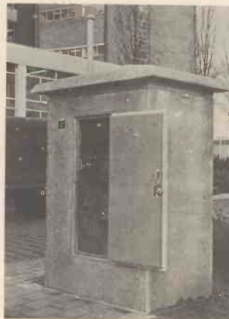
3. Monitoring cubicle for up to nine modular units.
