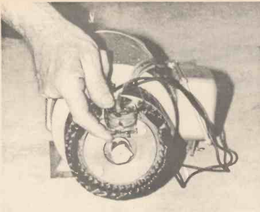
Coil imprints 'pole pattern' on magnetizable rotor.
