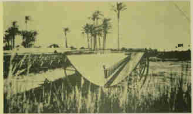
A solar collector built in 1913 and used beside the Nile River.
