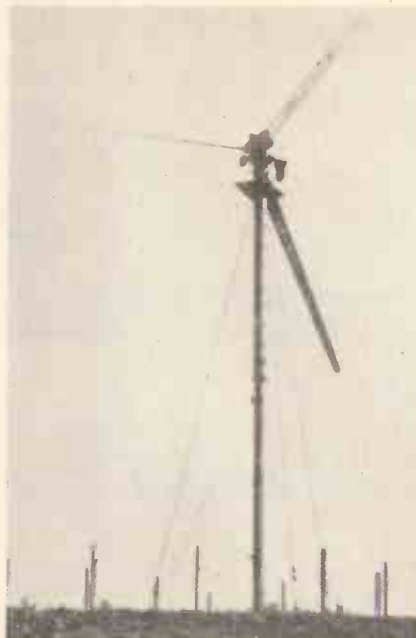
8 kw Allgaier experimental windmill built to supply an isolated croft in the Cairngorms, Scotland.
