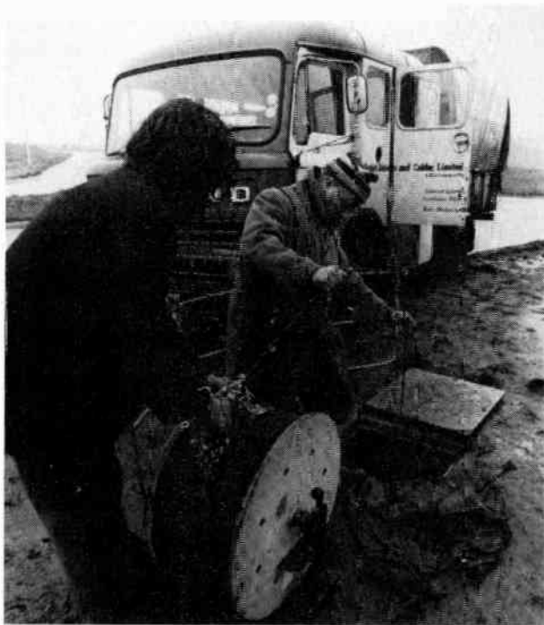
Fig. 1. Landline optical cable installation.
